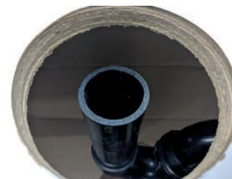
4. Apply glue to the outside of the ABS or PVC 1 1/2" pipe and to the inside of the P-trap.
