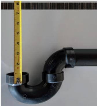
2. Measure the distance from the inside of the P-trap to the top of the floor.
