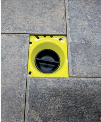
9. Install your flooring surface around the **opening** of the Drop-In Drain.
