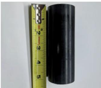
3. Cut the ABS or PVC 1 1/2" pipe **3 inches shorter** than the distance between the floor and the P-trap.
