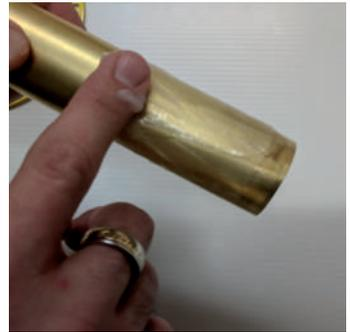
13. **Apply provided lubricant halfway up the tailpiece** and position the bathtub and tailpiece **in line** with the Drop-In Drain.
